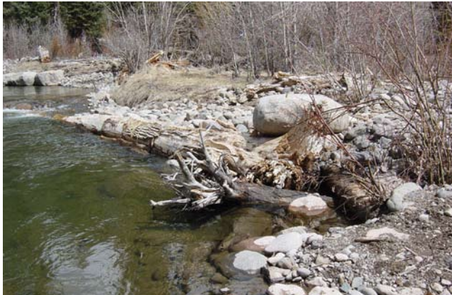
Figure 11-38 Rootwad/log vane/J-hook structure, East Fork Piedra River, CO
