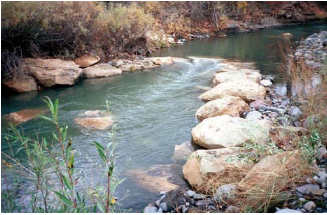
Figure 11-28 Cross vane installed on the lower Blanco River, CO
