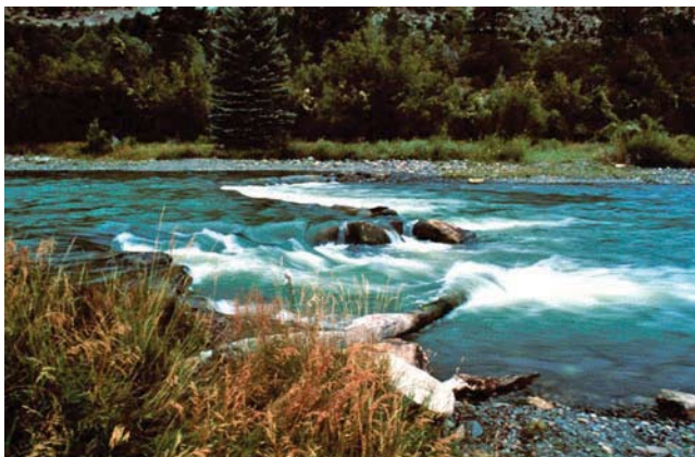
Figure 11-33 W-weir installed on the Uncompahgre River, CO
